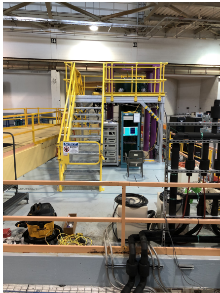
Shielding and stairs to upper detector in 2019
